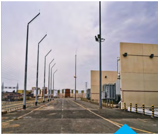
POWER PLANT PROJECTS KSA
